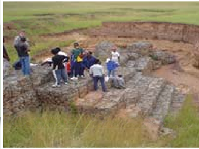
Beneficiaries construct gabion structures
